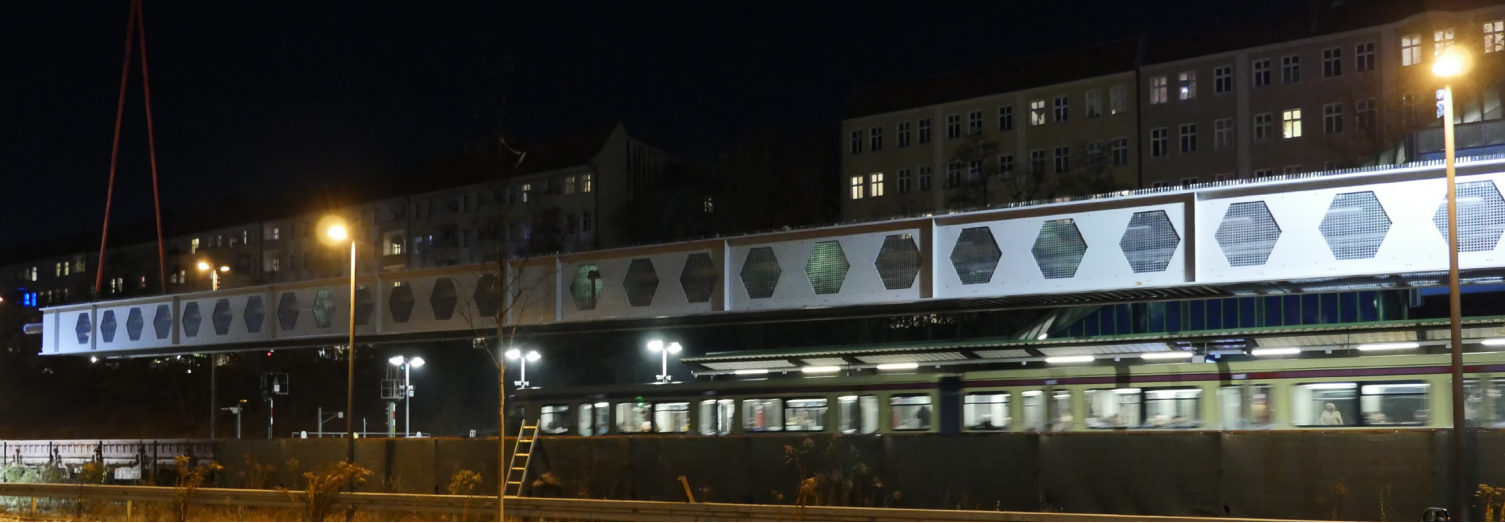
Final installation of a pipe bridge over DB Netz AG's railway system (©IBG)
